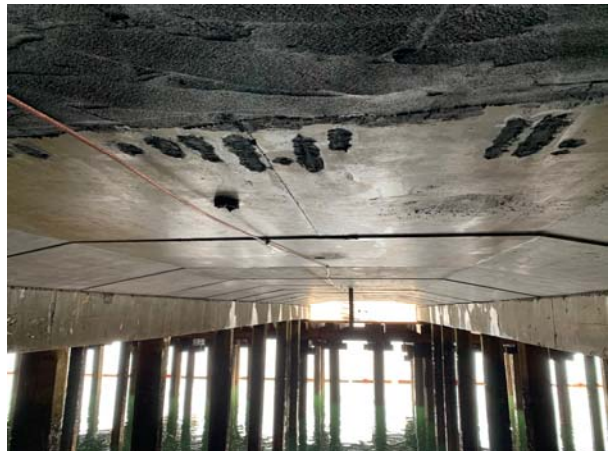
Under wharf repairs
