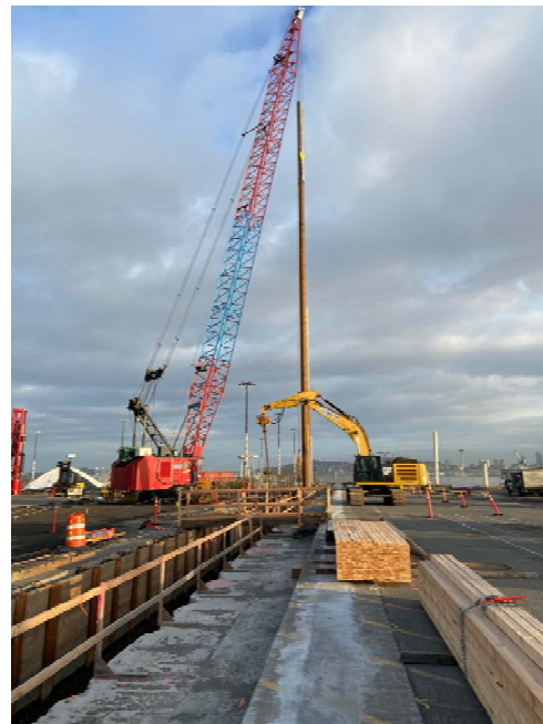
Landside Crane Rail - Drilling into the casings before vibrating the piles
