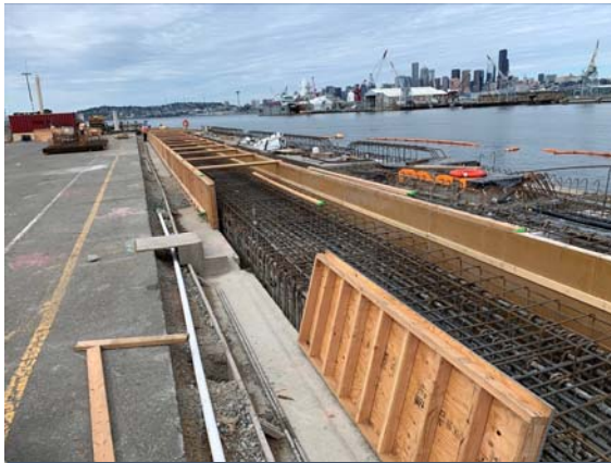
Waterside Crane Rail
